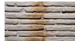
9- Waiting for drying for assembly putty
