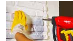
4-a) Assembling by nails
