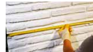
2- Scaling of the panel to be applied
