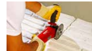
3- Cutting the panel by angle-grander
